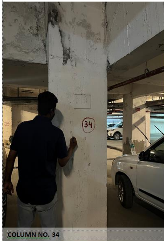
Images of Testing at Site:
